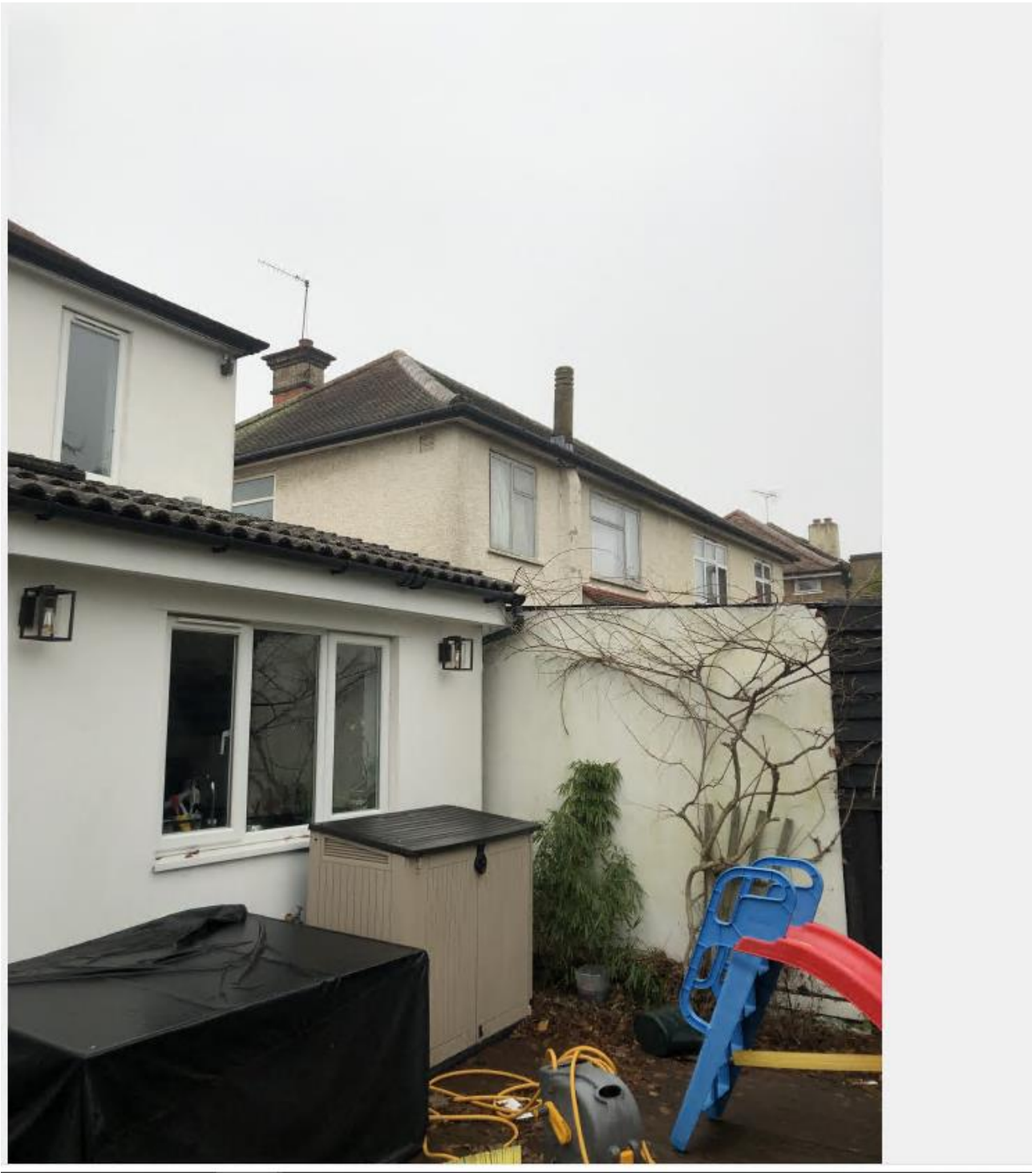
View of No. 33 from host property garden
