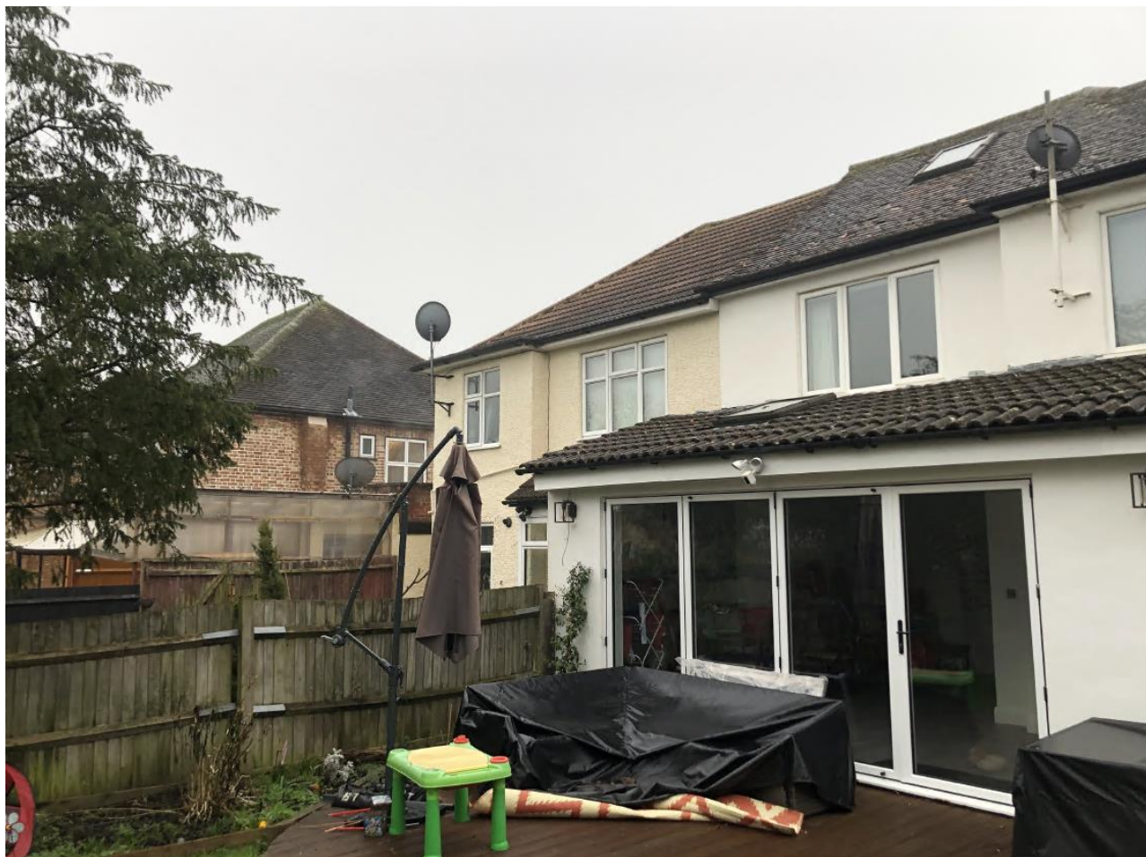
View of No. 35 from host property garden
